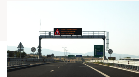
Bulgaria, motorway network
