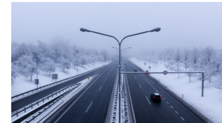
Czech Republic Road weather national system
